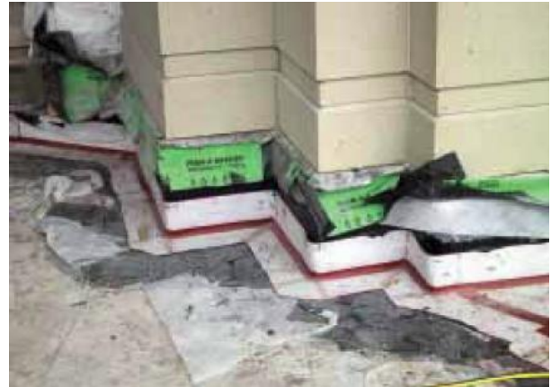
RedLINE 20G installed in Hot Rubberized Asphalt.
