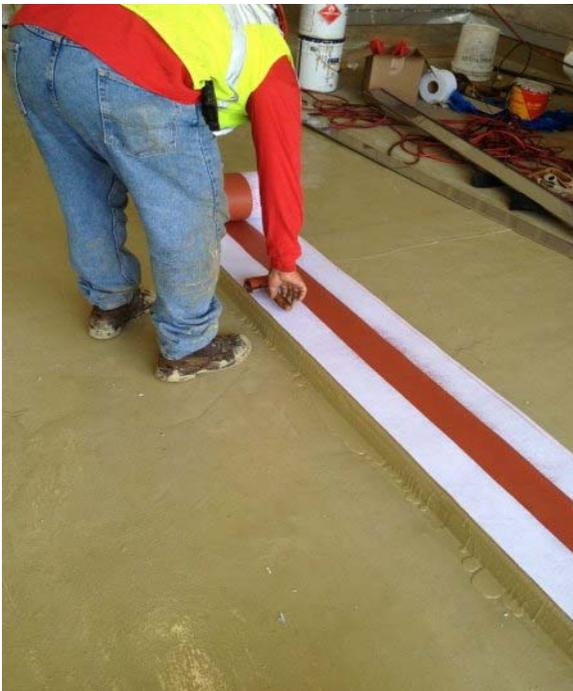
RedLINE being rolled to ensure proper adhesion
