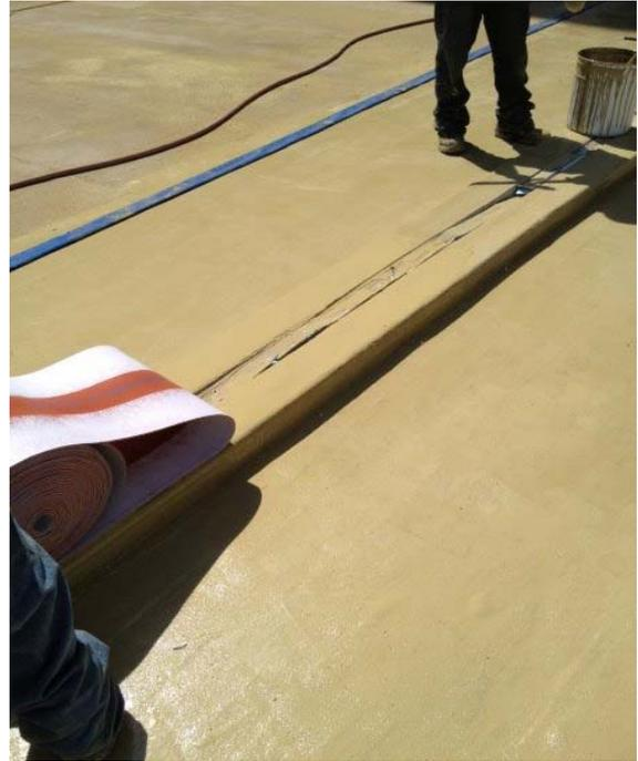
A coat of liquid membrane is being applied to the substrate
