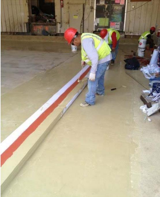
RedLINE fleece is being completely encapsulated and covered
