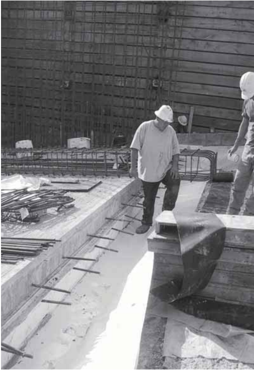
▲ The FlamLINE is being unrolled and installation.
