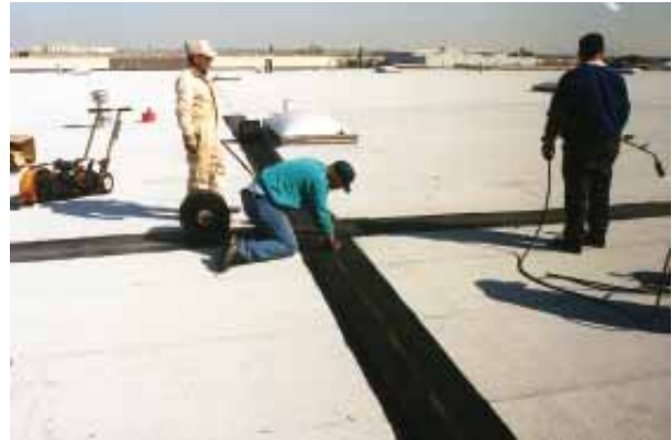
FlamLINE 100 installed in a torched system.
