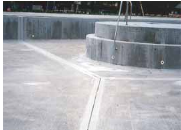
AquaLINE installed in potable water storage tank.
