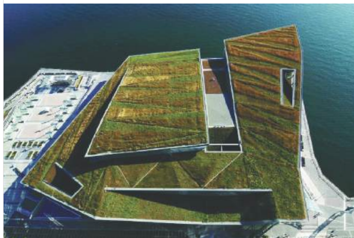
Vancouver Convention Center features Canada's largest living roof which is irrigated with wastewater from the building's own treatment plant.
