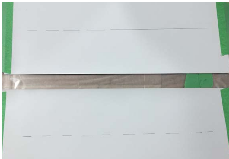
◀ The membrane with guide lines showing the extent of the RedLINE selvage edges, prior to any liquid membrane application.
