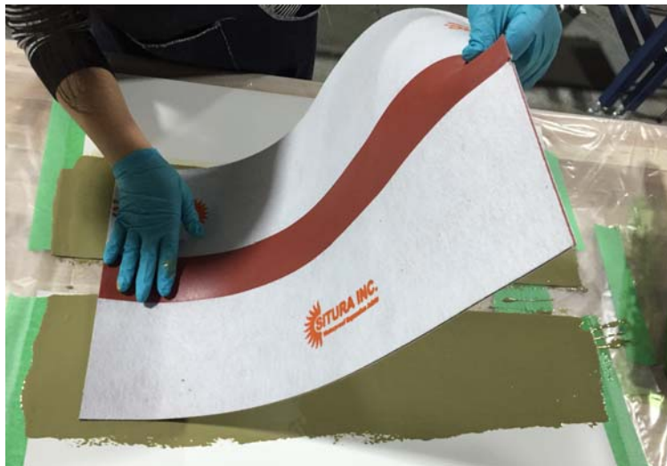
◀ The RedLINE expansion joint laid into the Kemper liquid membrane, Note; centering the RedLINE gland over the joint gap.
