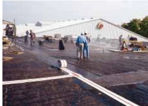
RedLINE 20 being installed in BUR.
