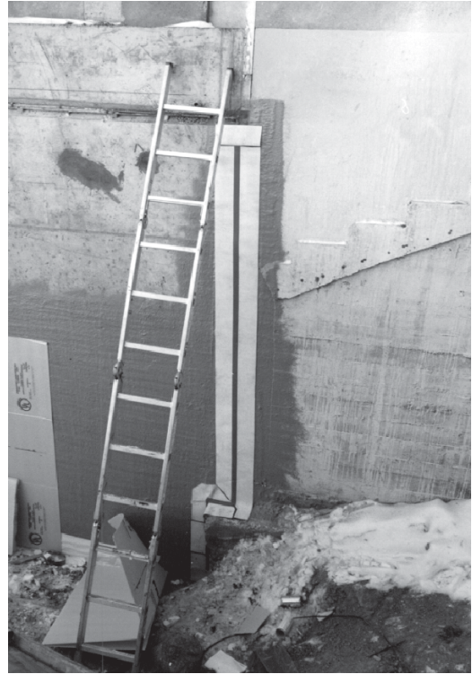
▲ The RedLINE joint is laid into a bed of freshly sprayed polyurethane.
