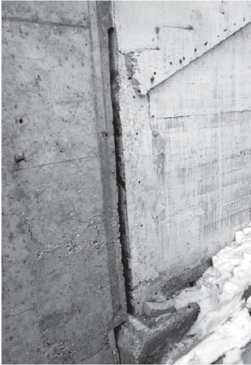
▲ An expansion joint gap at a foundation wall.
