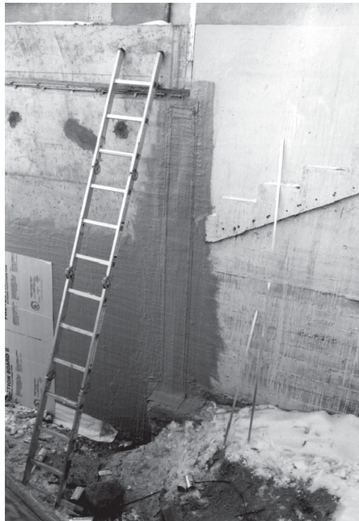
▼ The completed RedLINE installation in a sprayed polyurethane material.
