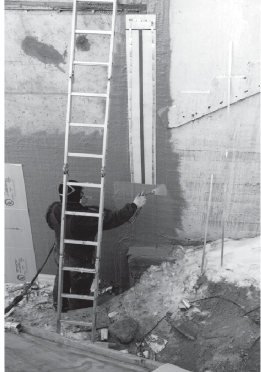
▲ The RedLINE being covered with the polyurethane.
