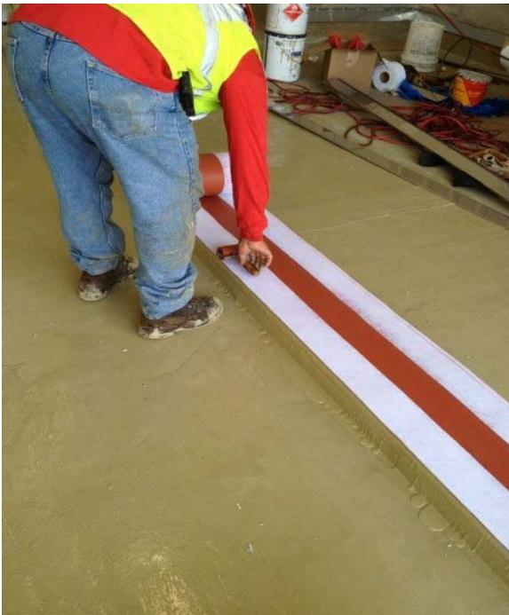
RedLINE being rolled to ensure proper adhesion
