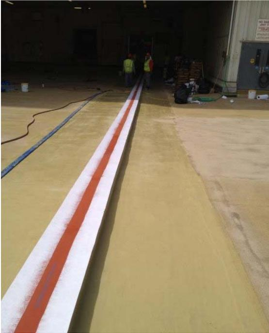
RedLINE being dry fitted to ensure correct fit
