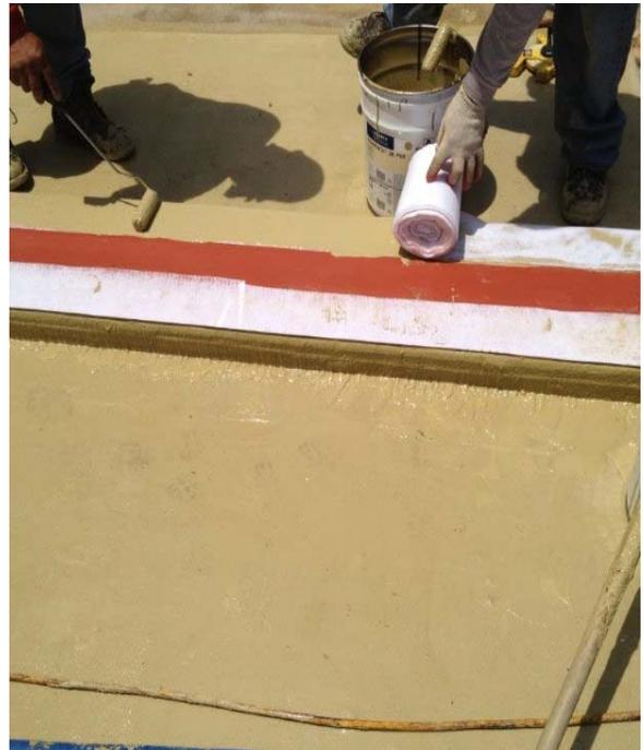
A coat of liquid membrane and the reinforcing fabric is being applied to the top RedLINE fleece
