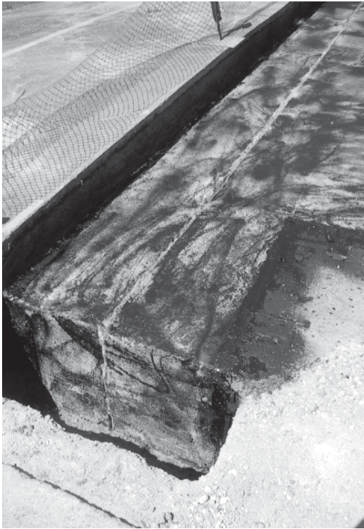
▲ The cleaned expansion joint cavity and primed concrete substrate.
