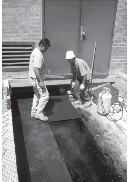
▲ The protection board being installed over the joint shingle fashion.
