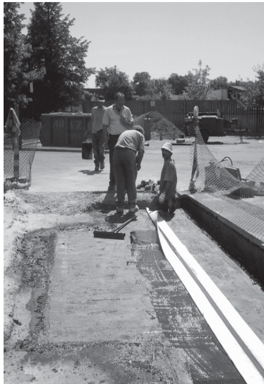
▼ The RedLINE is being rolled out into the hot asphalt.
