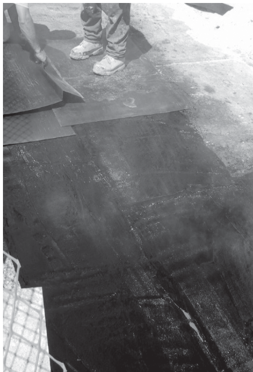
▼ The completed installation.
