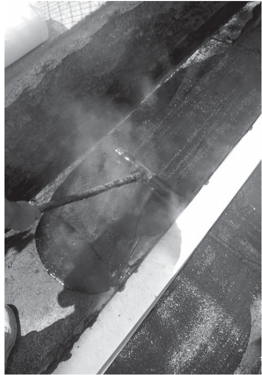
▲ Applying hot asphalt onto the concrete substrate.
