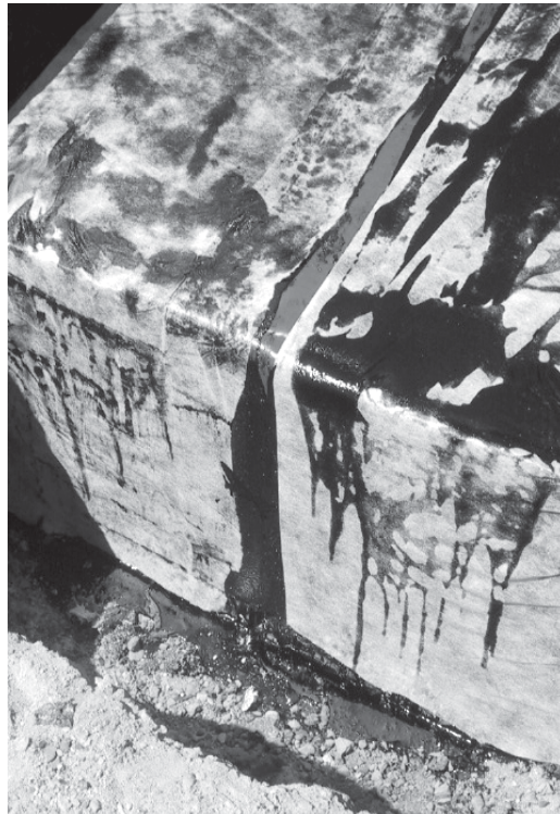
▼ The applied reinforcing fabric, note the RedLINE gland is not covered.
