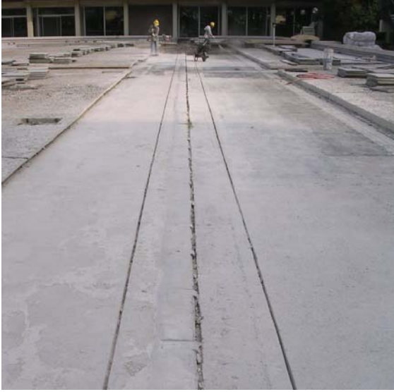
Substrate being prepared for epoxy application
