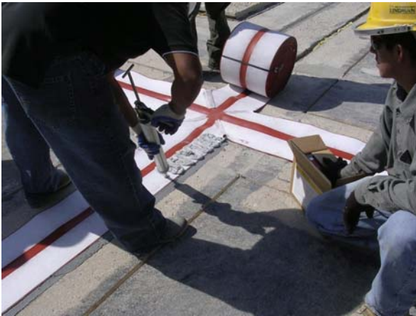
Epoxy is being applied to the top RedLINE fleece
