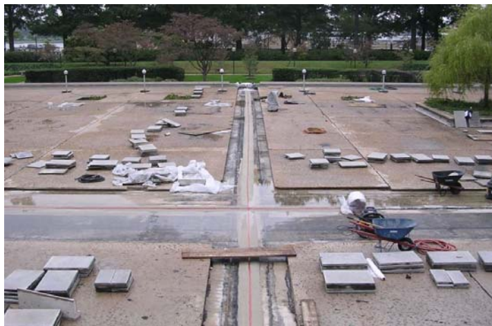
The completed RedLINE expansion joint installation
