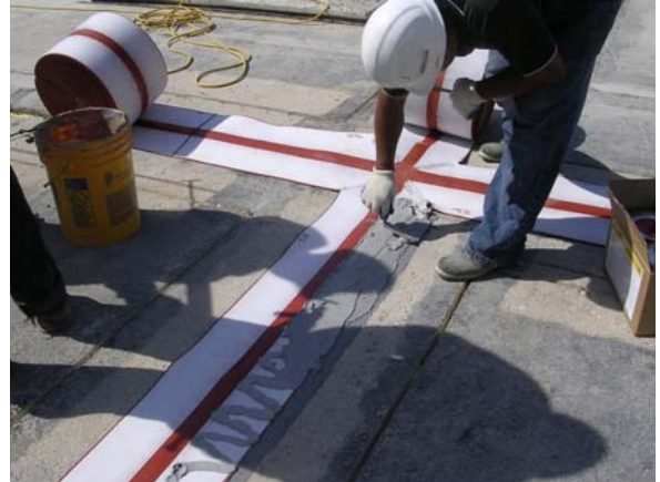
RedLINE is being encapsulated with epoxy
