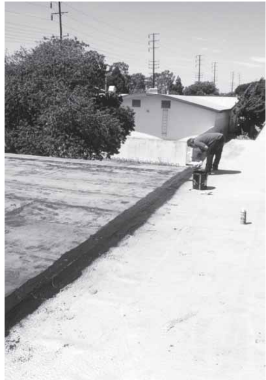
▼ The top side of the RedLINE is coated with the cold adhesive to provide waterproofing continuity.
