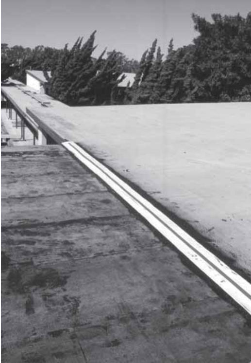
▲ The RedLINE is embedded in the cold adhesive bed.
