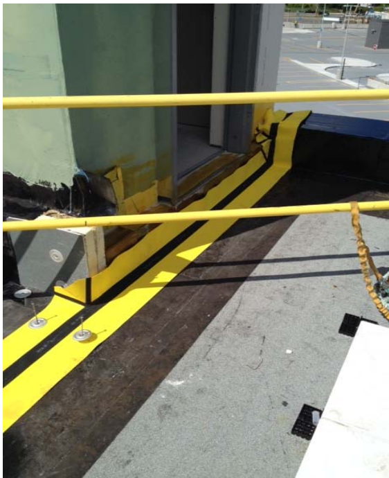
FlamLINE being dry fitted to ensure correct fit.
