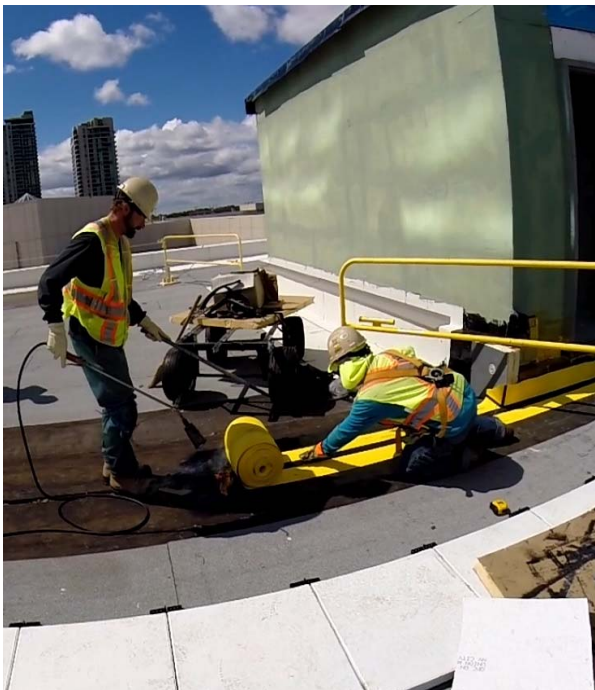
FlamLINE being adhered by rolling into liquified base sheet.
