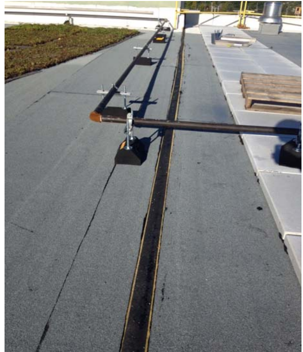
The completed FlamLINE installation
